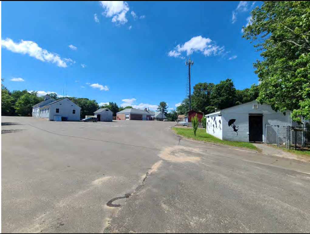
PHOTO NO. 5 DESCRIPTION: View of the drainage area from rear parking area; dog pound, rear of emergency management building.
