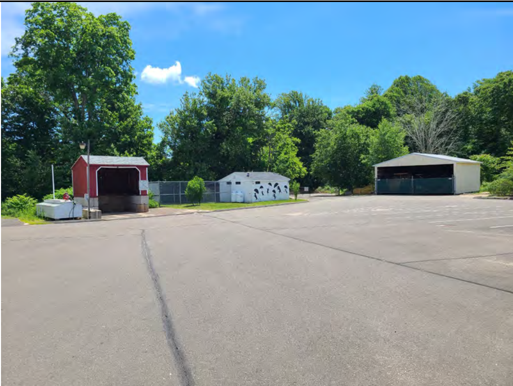
PHOTO NO. 4 View of aboveground storage tank, sheds, and dog pound. DESCRIPTION:
