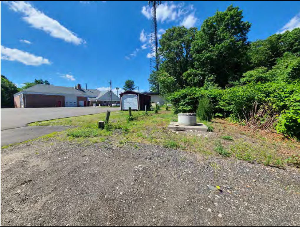
PHOTO NO. 3 View of the cistern access/location, shed, rear of fire station. View of the former fire training area to the left of photo. DESCRIPTION:
